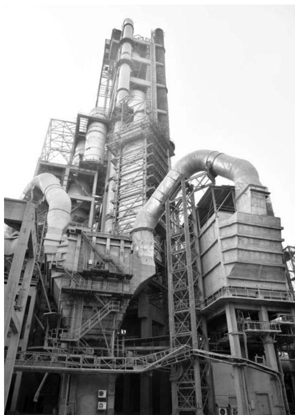
5 stage Pre Heater and Electrostatic Precipitator (ESP)
